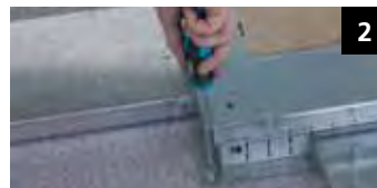
Insert the trunking and screw to floor
