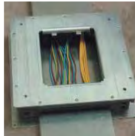
Trim cover for flush-mounting
